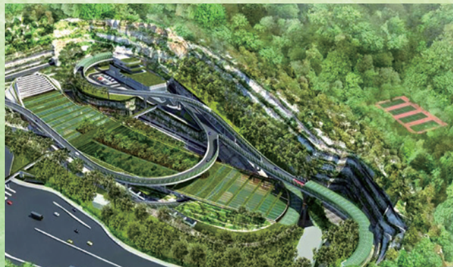
Tseung Kwan O — Lam Tin Tunnel and Related Projects
