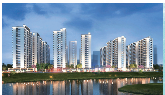
Government Targeted Repurchase Project (Plot 04-B-29), Innovaland, Lucheng District, Wenzhou, Zhejiang Province
