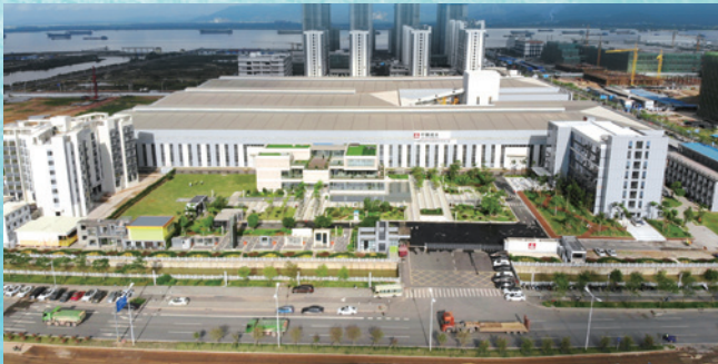
Zhuzhai Hailong Construction Products Plant
