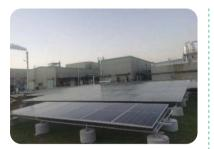
Wenling Solid Waste Treatment Project has constructed solar energy facilities at locations such as rooftops of the plant buildings, accident pools, preliminary rainwater captures with an installed area of approximately 12,000 m<sup>2</sup>, and an aggregate installed capacity of approximately 1.6 MW.
