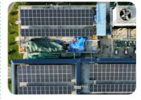
Linshu Hazardous Waste Incineration Project utilises the existing building space of the plant site to install solar energy facilities at the common engineering building, integrated pump chamber, mechanical repair workshop and laboratory, respectively, occupying an area of approximately 2,000 m<sup>2</sup> and providing installed capacity of 0.4 MW.
