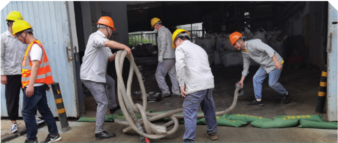
Special drill for flood prevention and drainage
