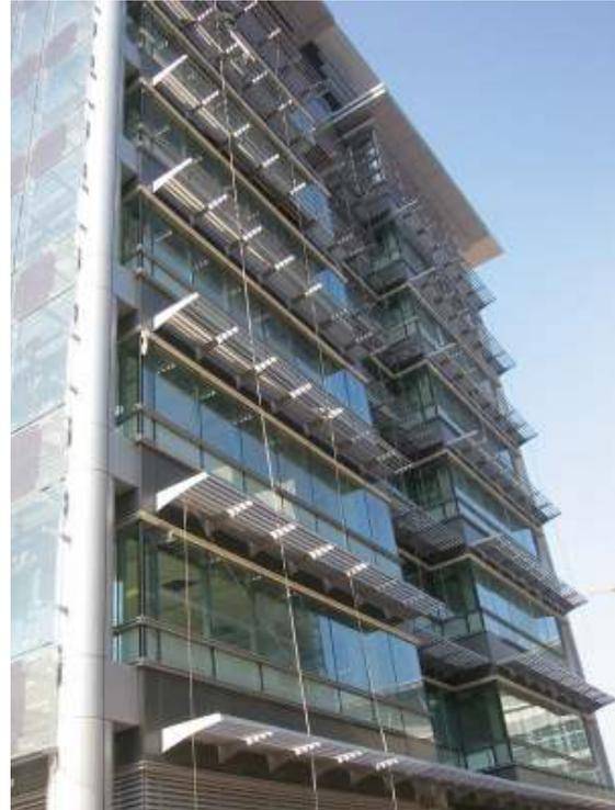
Sun shades are used to shield a building from excess sunlight and help to improve the energy efficiency of a building by reducing the amount of air conditioning required in the building.
