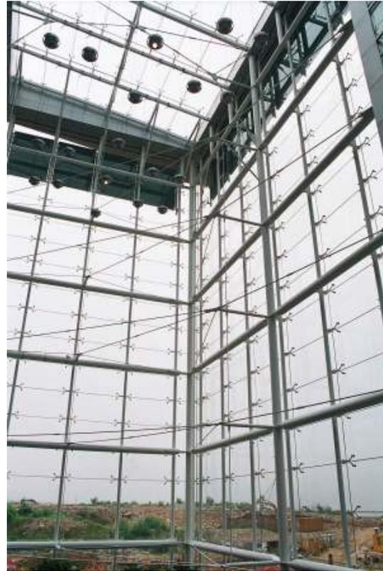
Glass walls are generally used in the podium, lobby or atrium portion of a building where the floor height is higher than the other floors of the building. Glass walls can be supported by steel frames, aluminium frames and other structural materials and are typically not used as the facade of the individual floors of a building. Shopfronts are generally constructed by glass panels supported by structural frames to enhance the attractiveness and transparency of retail shops.
