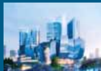
SHANGHAI Xinzhuang Metro Superstructure
