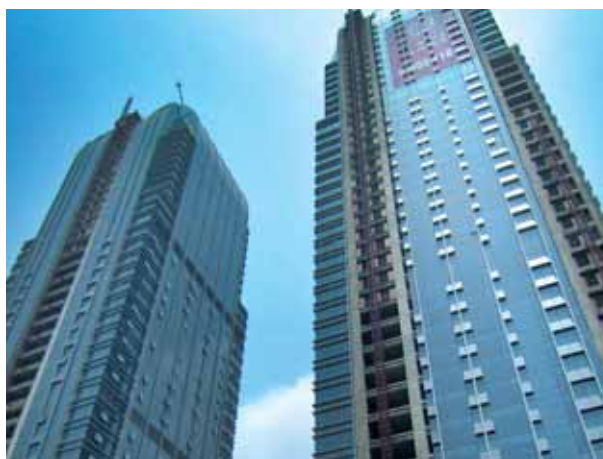
Urban Development International Centre—Under development
